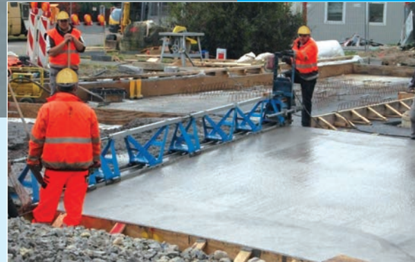
Road-building with the NOGGERATH Variant® - 2.2
