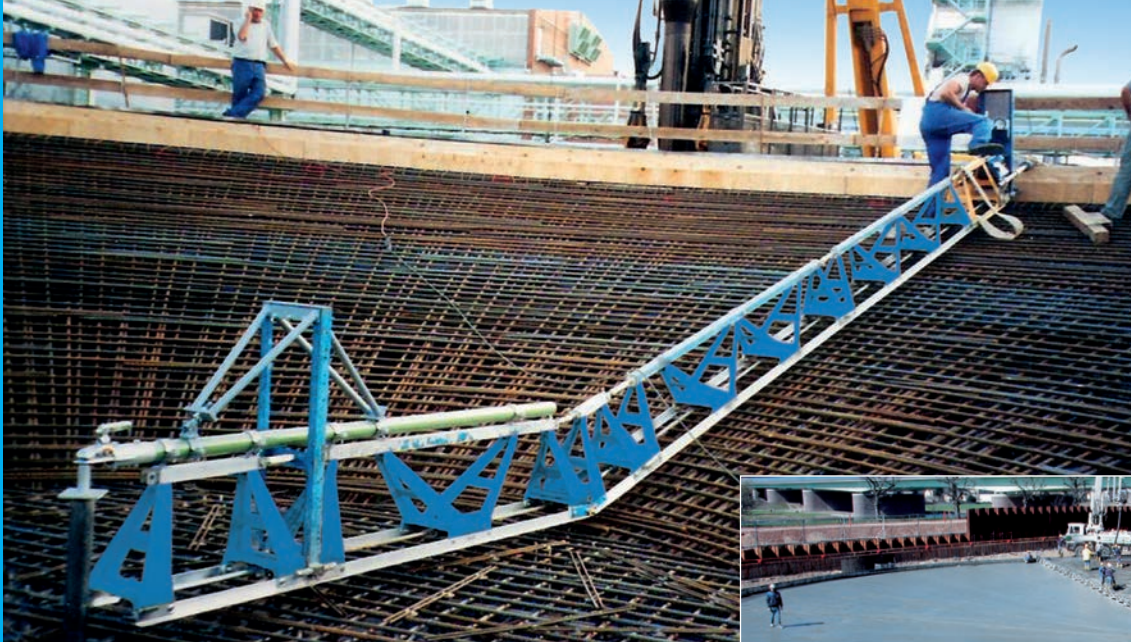
Concreting with break-point
